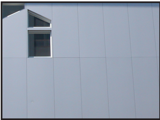
Invisible fixing gives panelling a smooth appearance.
