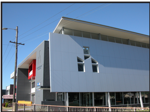
MBA Building in Newcastle.
